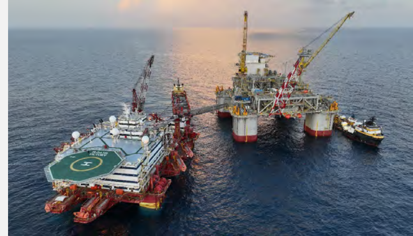
Floatel Victory alongside Chevron Anchor FPSO, US Gulf of Mexico
