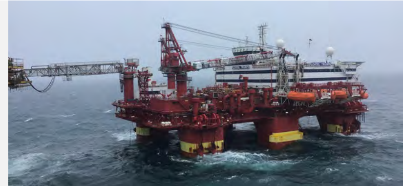
Floatel Triumph commenced operation on schedule at Shell Shearwater May 1, 2024, following completion of thruster overhaul, UK continental shelf
