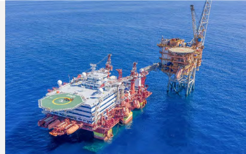
Floatel Triumph in operation for Woodside Pluto offshore Australia
