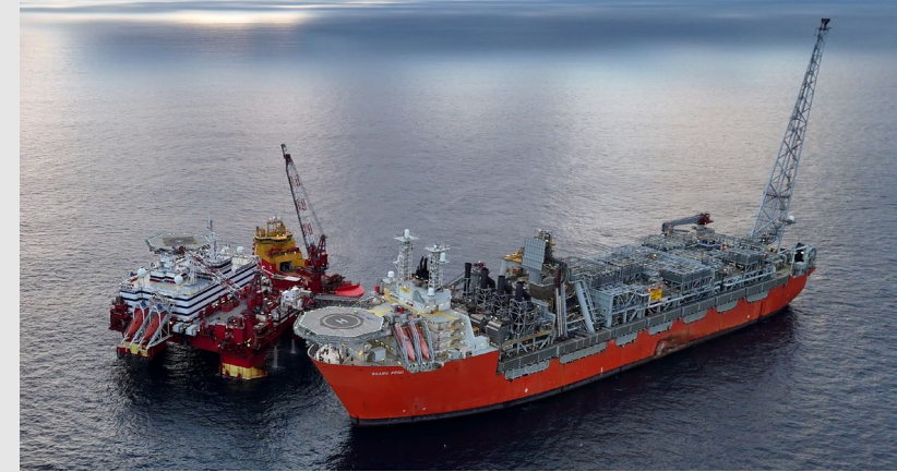
Floatel Endurance in operations for AkerBP at the Skarv FPSO, Norway
